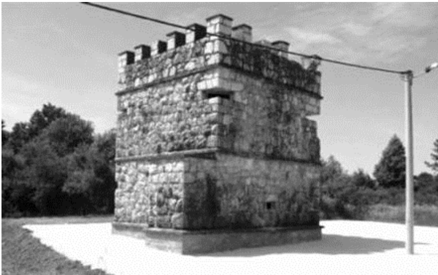
Figure 4. Renovated bunker in Karlovac
