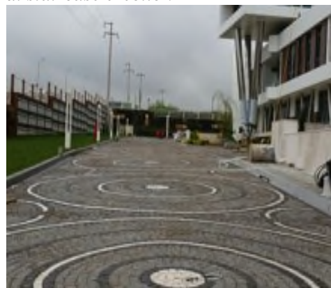
f. traffic facility construction
