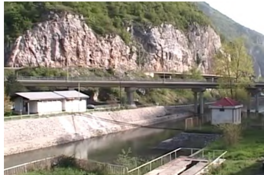
Figure 4. Pipe system for supply hot water from dug well (foto: Maja Obradović)
